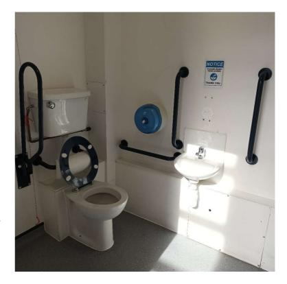
The sink, soap, toilet paper, and/or paper towels should be relocated to allow use whilst seated on the toilet.
